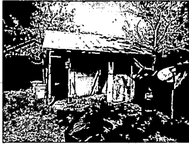
Shed in disrepair No Value
